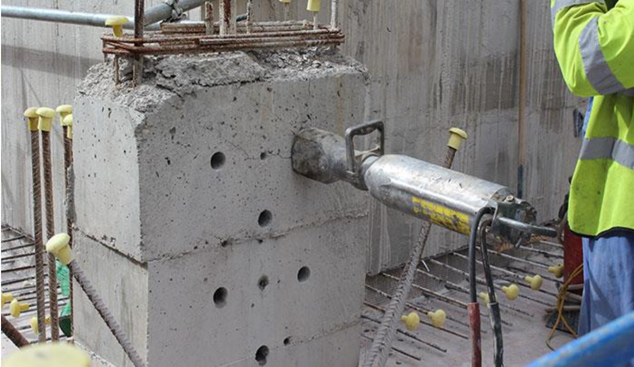
Fig.3 bursting concrete
